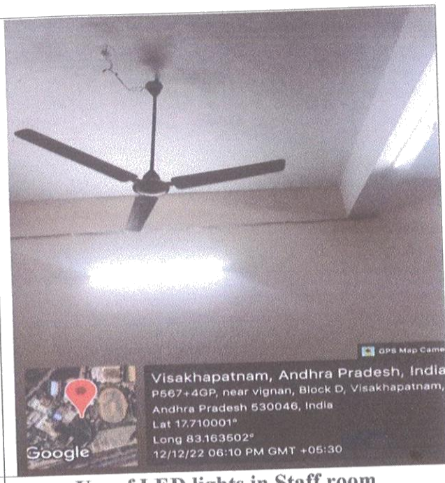
Use of LED lights in Staff room
